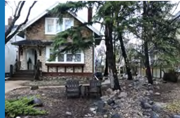
Image 86. Dry swale (image credit: Hazel Borys)
